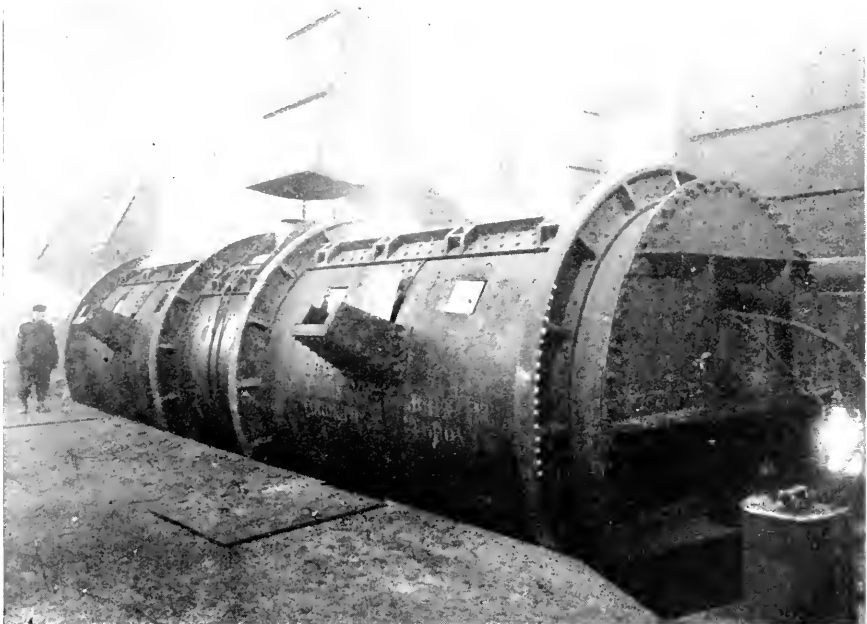
Fig. 73—Converter, Canadian Copper Company, Copper Cliff, Ontario.
